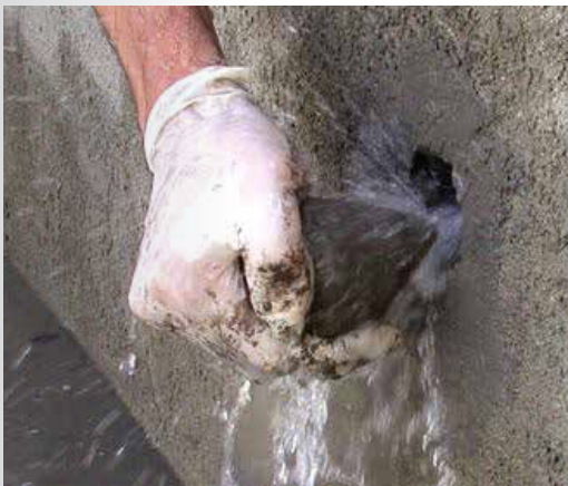
a) For plugging of active leaks;
